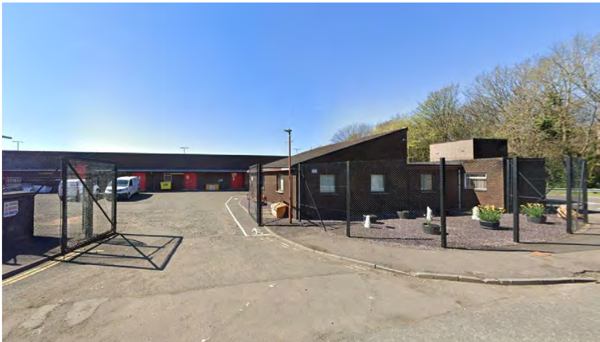
Figure 1: Image of the Estates Block
