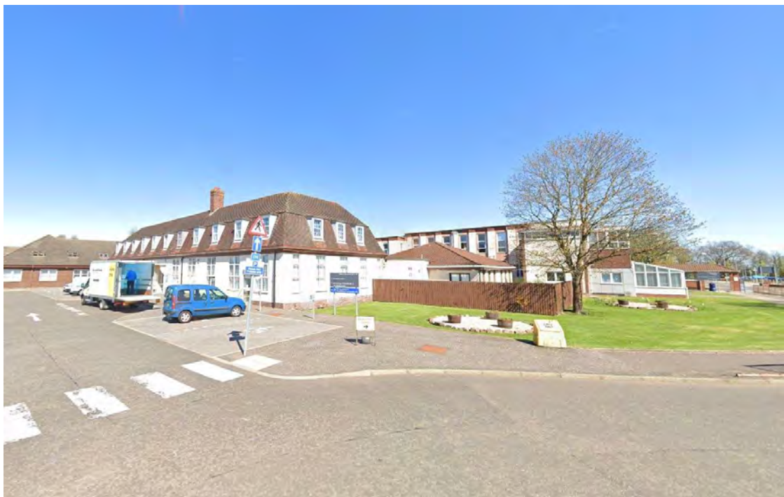
Figure 1 - Image of the Rehabilitation Ward, Stirling Community Hospital
