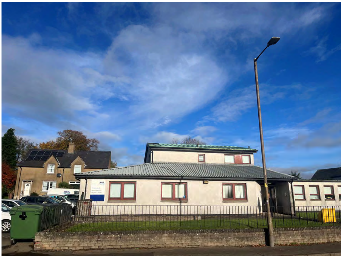
Figure 1 – Bannockburn Health Centre
