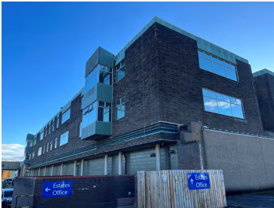
Figure 1 - Falkirk Community Hospital Surgical Block
